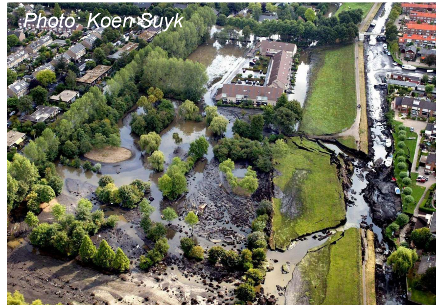
Failure of the Wilnis levee in the Netherlands, August 26, 2003
