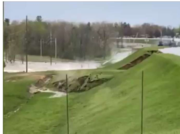
Edenville dam collapse, May 2020 (YouTube video by Lynn Coleman)
